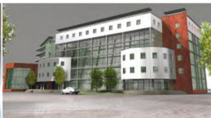
Saadi Shiraz Commercial Office Complex
