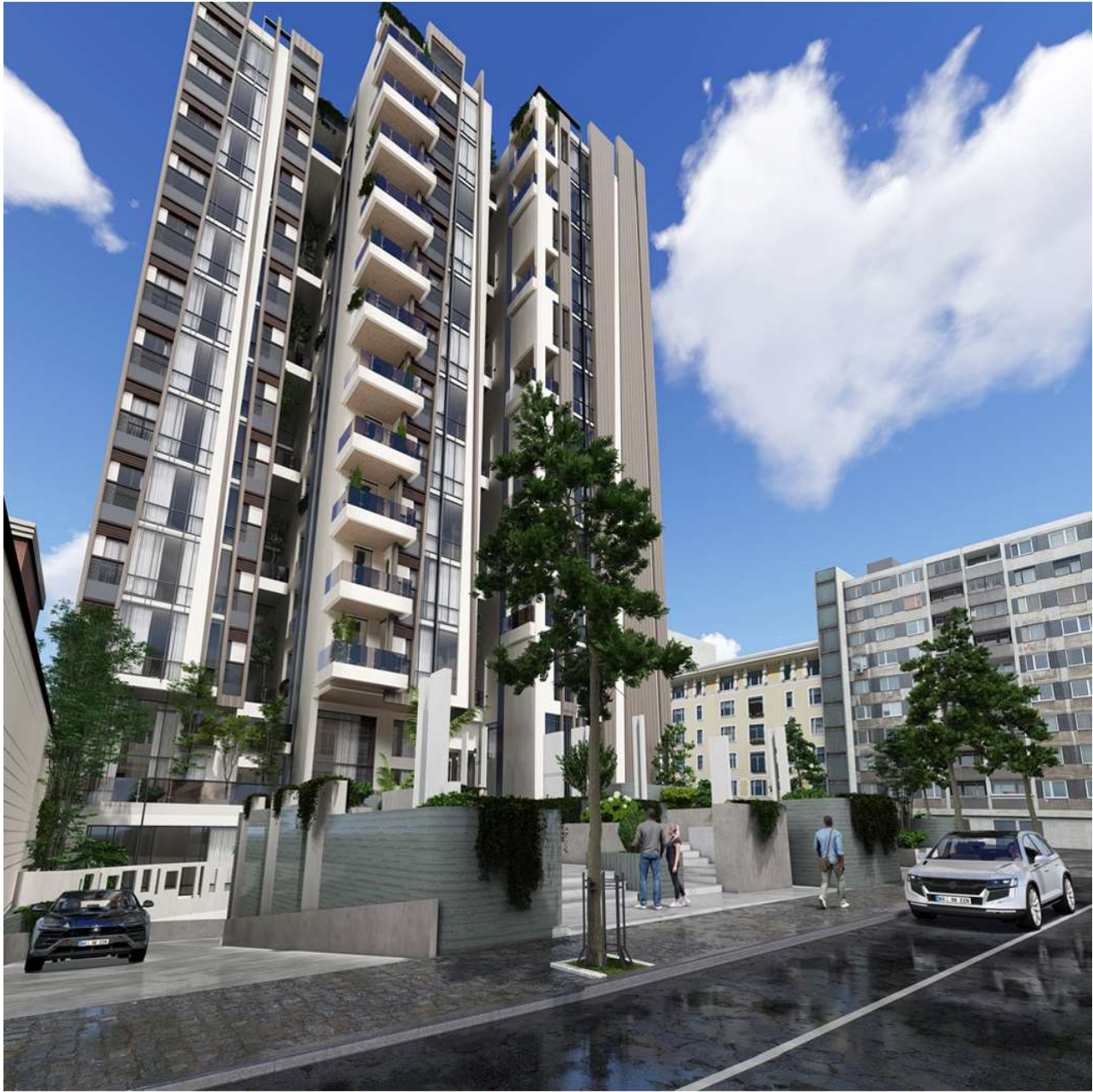
South-West Side's General View ,
