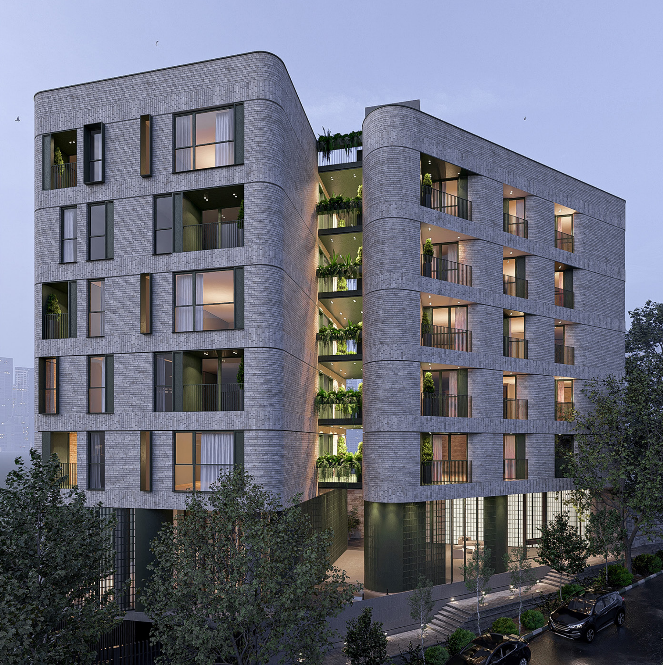
South and East Facade
