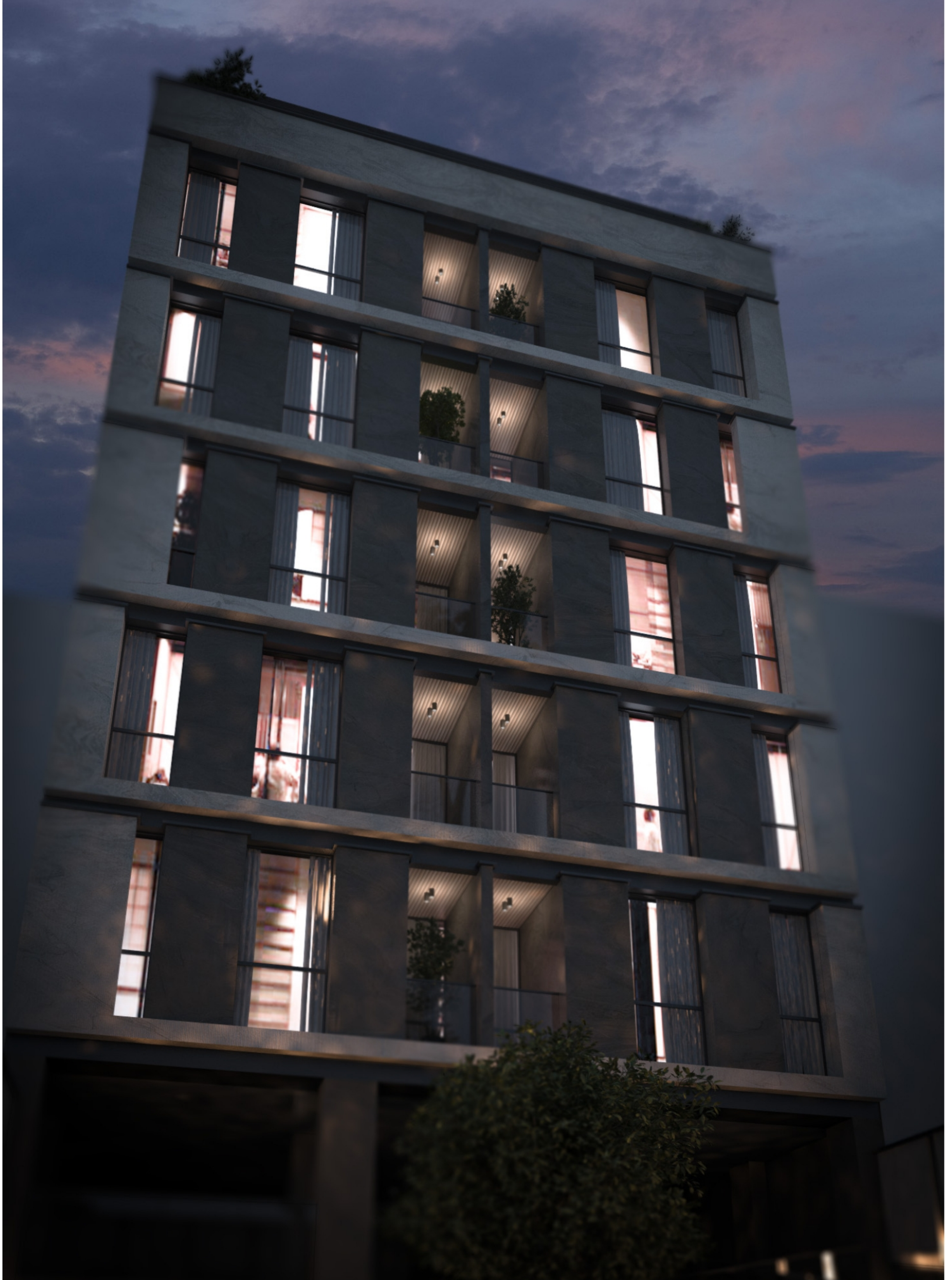
SOUTH FACADE (LIGHTS)
