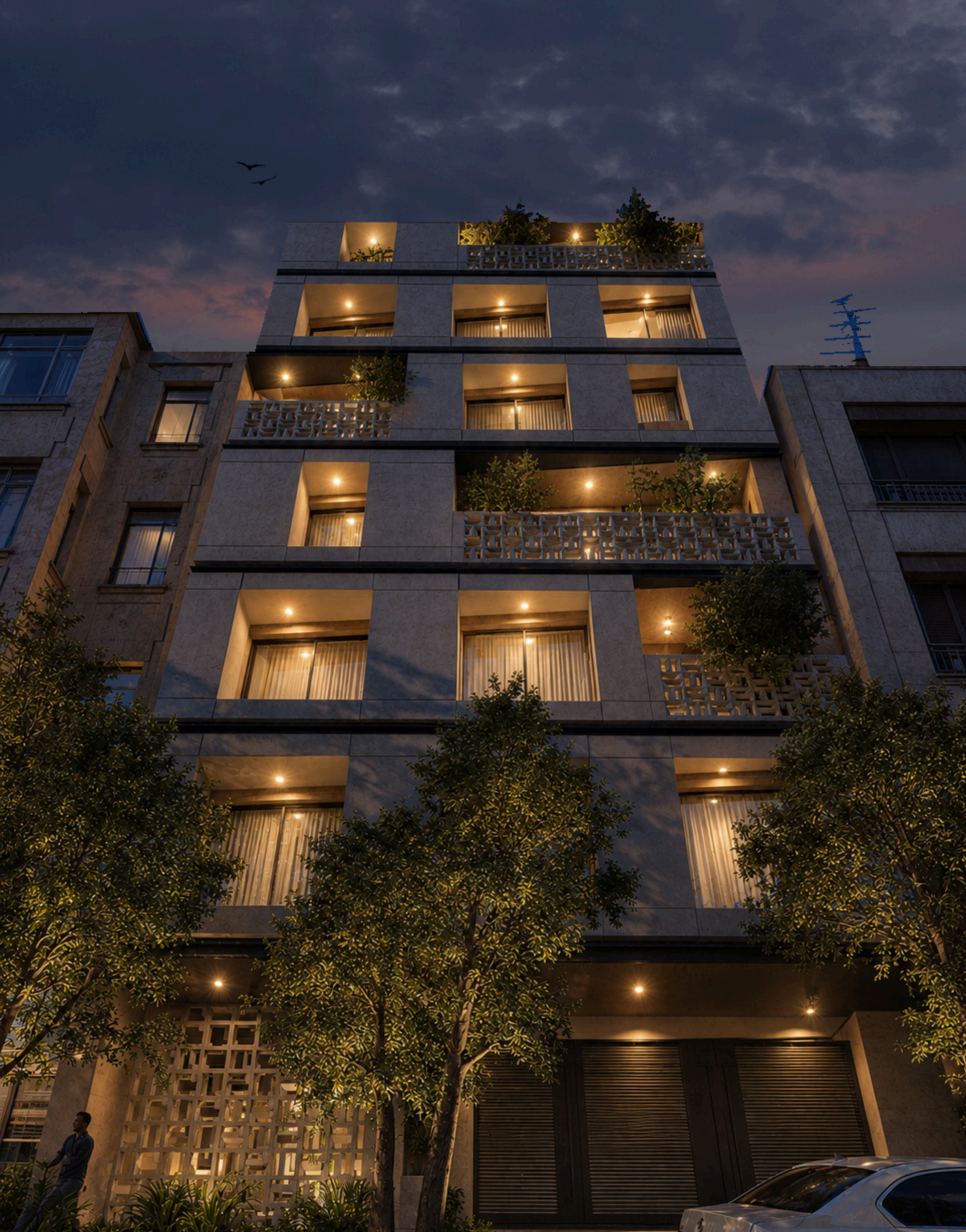
NIGHT NORTH FACADE
